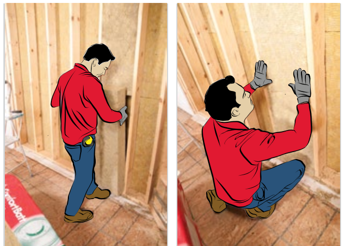
ROCKWOOL Comfortbatt® higher density batts make it simple for precise cutting to ensure a fit without gaps and voids.
